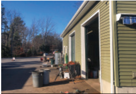
Side view of Shop/Storage
