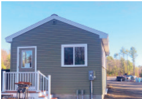
Office Building/Scale House
