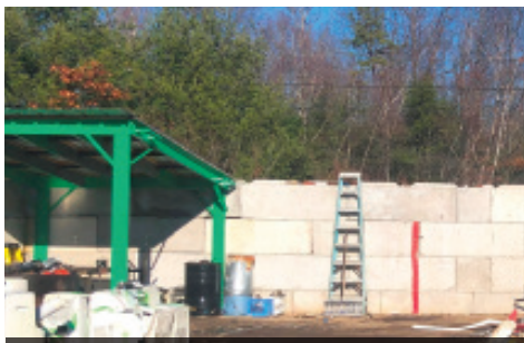
Slab with Containment Block Walls
