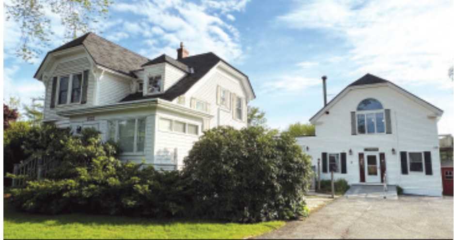
MAIN BUILDING AND CARRIAGE HOUSE
